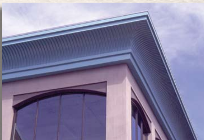
Office Building Cornice System
