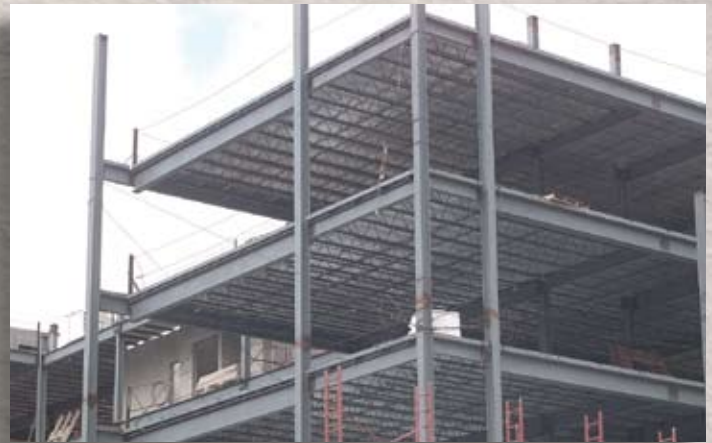
9/16" Form Deck on Bar Joist
